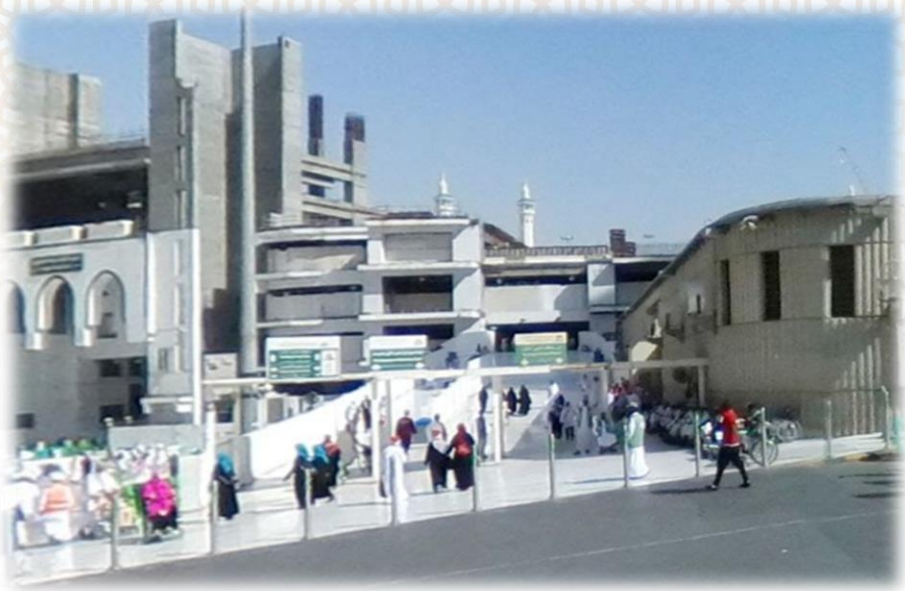
Figure 3 - Ramp up to first floor
