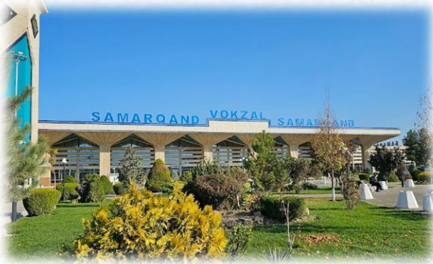
Figure 30 - Samarkand Railway Station
