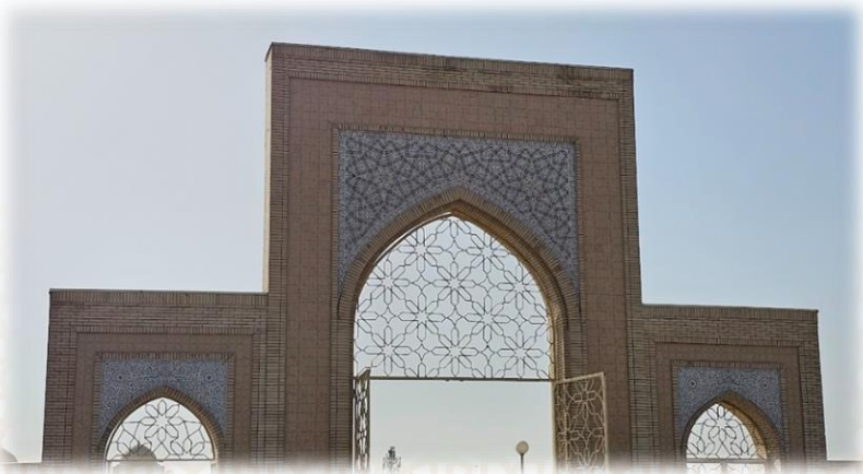
Figure 48 - Entrance to complex
