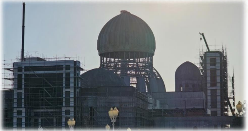
Figure 3 - New Masjid at Imām Bukhārī رَحْمَةُ اللَّهِ complex
